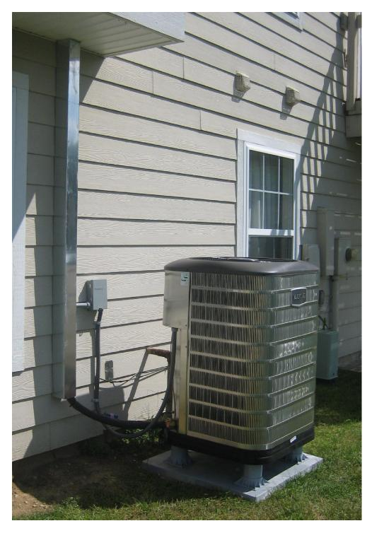
Picture One - Installation example: Removal of the old mounting bracket and replacement with a purpose-made pad is acceptable. The length of the new refrigerant lines (in chase) is acceptable. The metal chase itself (not paintable) is not acceptable and must be replaced.
